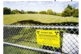
Approximately 300 locations in Port Hope have been identified as contaminated by the uranium industry.
